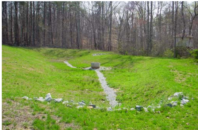
Example of a dry detention basin.
