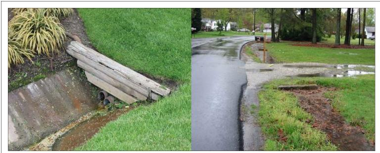
Drain blockages can be natural or man-made. At left, a property owner has illegally covered a ditch and put in pipes that are too small to adequately handle the amount of water the ditch was designed to handle. At right, a collection of leaves has bunched up in front of a pipe, blocking water from getting through.
