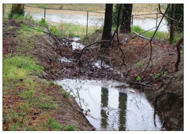
Tree branches and leaves are a common cause of storm drain blockages that can contribute to flooding during heavy rains.
