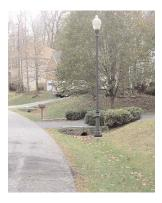
**Grass swales** are an alternative to the curb and gutter system. Grasses or other low-growing vegetation are planted to reduce runoff velocity and allow filtration, while high-volume flows are safely channeled into a storm sewer or retention basin. Native plant species such as white ash, red cedar, chokeberry, sunflowers and switch
