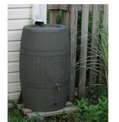
Stormwater can be collected from rooftops by diverting downspouts into rain barrels. Rain barrels help slow the flow of runoff from impervious surfaces and store water for future landscape uses. Multiple rain barrels can be linked together to increase storage capacity.
