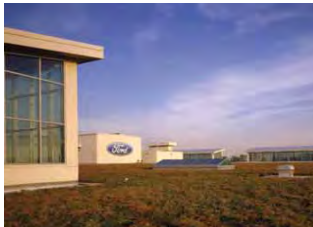
At more than 10 acres, the largest green roof in the world sits atop Ford's Rouge River Manufacturing Complex. The green roof is one component of a renovation designed to make the facility more environmentally sustainable. PHOTOS COURTESY OF GREEN ROOFS FOR HEALTHY CITIES
