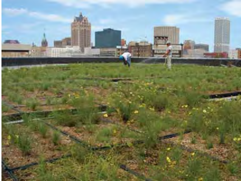
The green roof atop MMSD's headquarters, shown just after installation, demonstrates how stormwater flow into the city's sewer system could be reduced.
