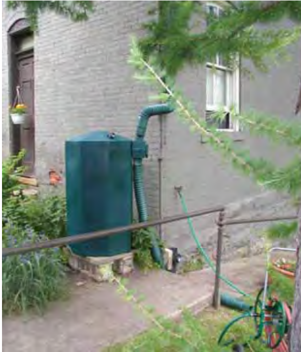
A RiverSafe RainBarrel installed at the Jane Holmes nursing residence in Pittsburgh, PA, by the Nine Mile Run RainBarrel Initiative.
