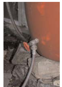
Open the water spigot and fully drain your barrel before the first winter's freeze.
