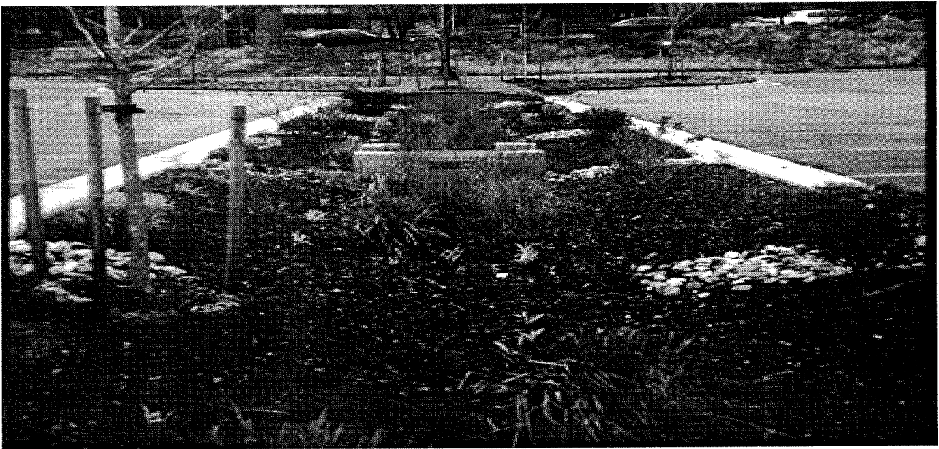
Figure 10.2: Bioretention Area (Prince Georges County, Maryland)
