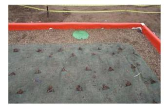
These assemblies are suitable for roofs with pitches less than, or equal to, 1.5:12. Large vegetated covers will generally incorporate a network of perforated internal drainage conduit.
