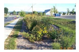
Subsurface Infiltration Beds provide temporary storage and infiltration of stormwater runoff by placing storage media of varying types beneath the proposed surface grade. Vegetation will help to increase the amount of evapotranspiration taking place.
