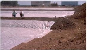
recommendations. Adjacent strips of geotextile should overlap a minimum of 16 in. It should also be secured at least 4 ft. outside of bed in order to prevent any runoff or sediment from entering the storage bed. This edge strip should remain in place until all bare soils contiguous to beds are stabilized and vegetated. As the site is fully stabilized, excess geotextile along bed edges can be cut back to bed edge.
