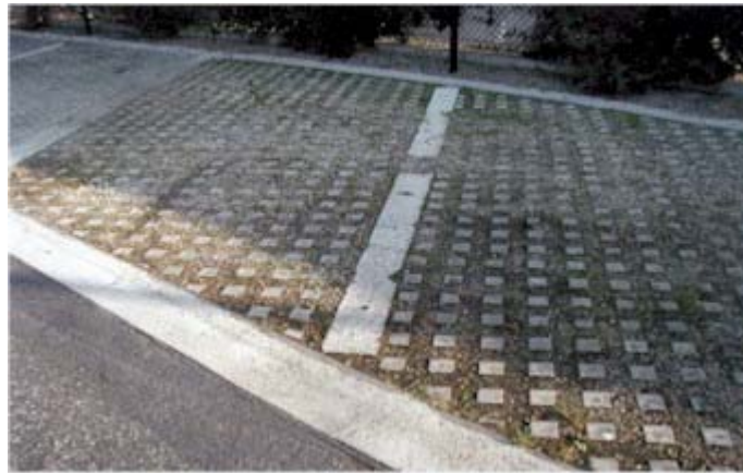
Figure 5.10-2 Overflow parking using permeable pavers
