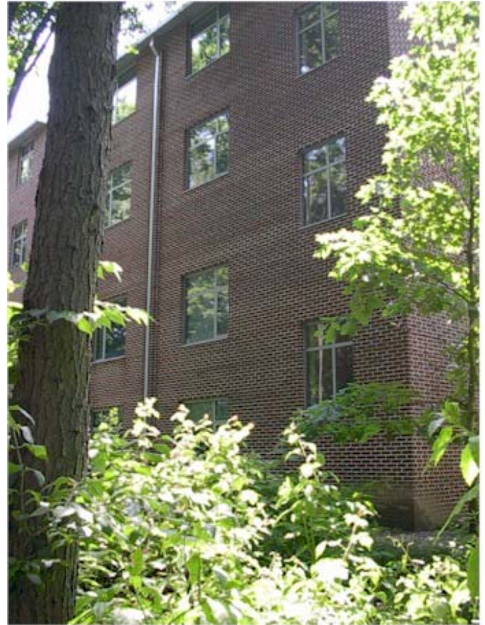
Figure 9-26. Example of minimum disturbance and prevent erosion or disturbance on the hillside.
