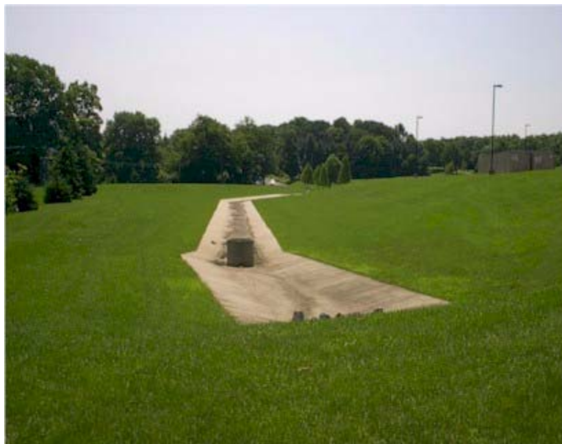
Figure 9-25. Existing sinkhole-plagued detention basin.
