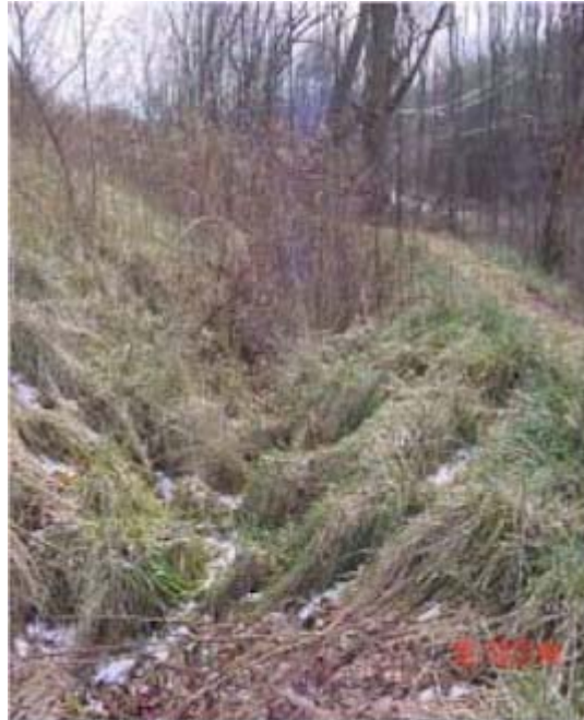
Figure 9-34. Narrow, vegetated infiltration trenches/berms follow land contours and take on a naturalized appearance.
