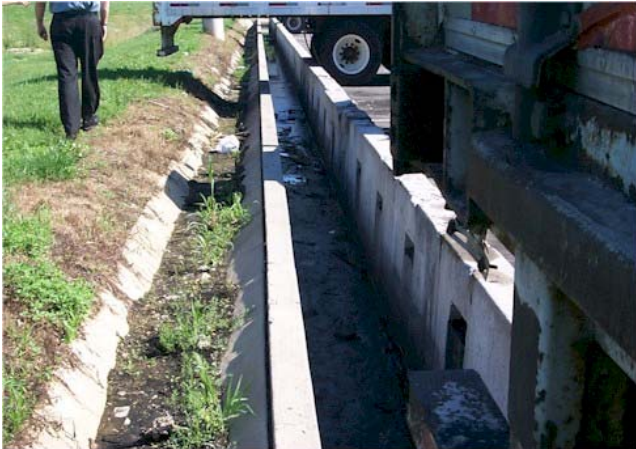
Figure 9-16. Perimeter trench drain.
