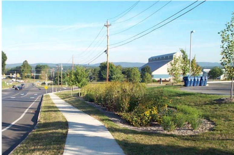
Figure 9-8. Porous concrete sidewalks, State College, Centre County.
