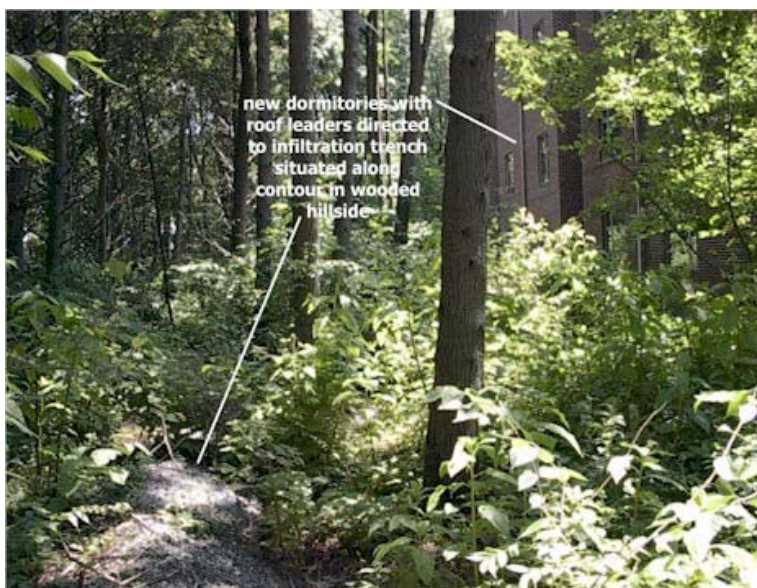
Figure 9-27. Level spreader pipe/infiltration trench in woods.
