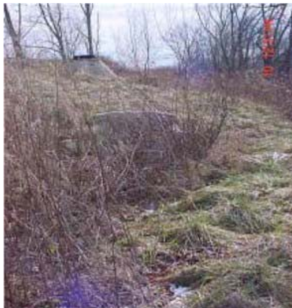
Figure 9-35. This trench/berm has a subsurface energy dissipater to reduce the velocity of entering stormwater.
