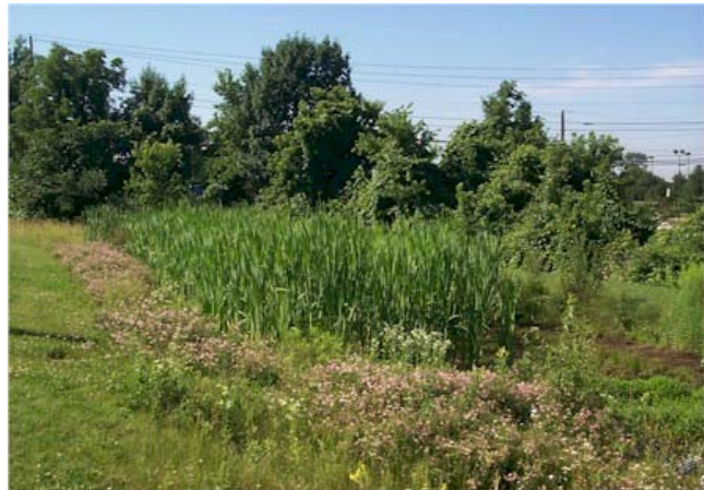
Figure 9-17. Vegetated infiltration filters.
