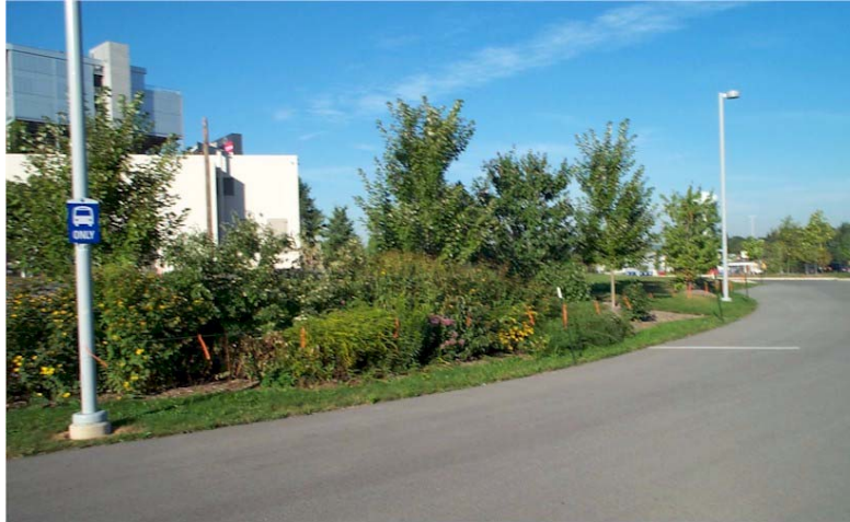
Figure 9-5. Vegetated infiltration bed, State College, Centre County.
